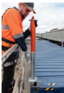
Place container post into ISO corner casting
