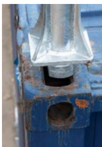
Place container post into ISO corner casting
