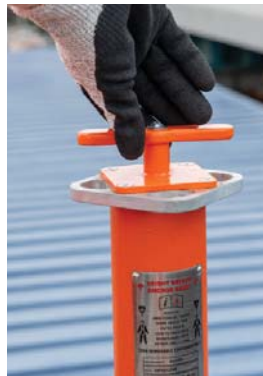
Rotate crank handle until firm
